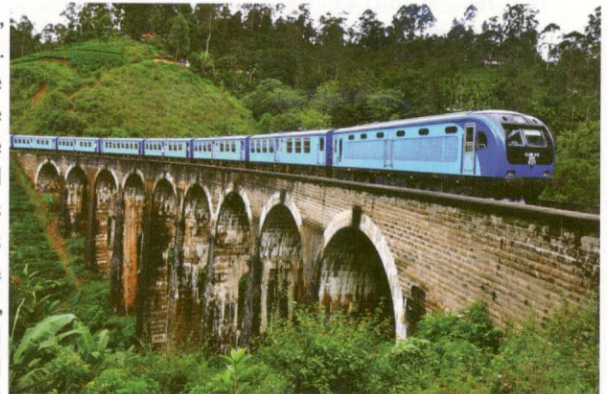
Latest Class S12 Diesel Multiple Unit with an Sifang diesel-electric locomotive each at the front and the rear, electronically synchronised passes over the Nine Arch Viaduct. The viaduct has withstood rail traffic for nearly one hundred years, including the heavyweight of the steam-era, the Beyer Garratt, without settlement.
